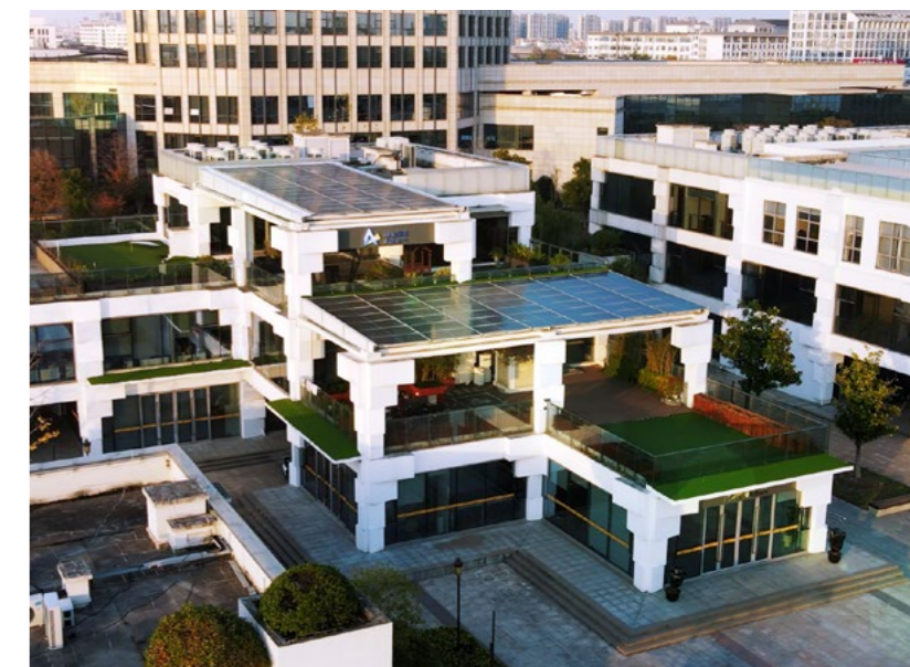
Roof photovoltaic project of AlphaESS Suzhou Branch
